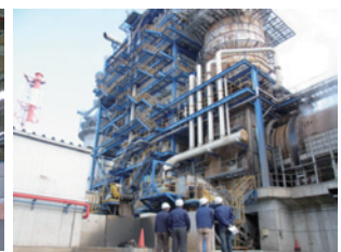
Field check of waste processing facilities (2013 Co. B)
